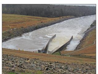
The Army Corps of Engineers, a part of the U.S. military, releases water from the dam at Jordan Lake, located at the Haw and New Hope rivers. Normal release flow is between 500 and 1,000 cubic feet per second. This release last week shows around 8,900 cubic feet per second, the equivalent of more than 66,576 gallons of water per second. (Staff photo by Zachary Horner)
